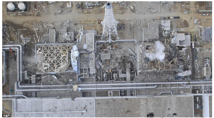
Fig. 2 Directly above the site taken photo on 20 th of March, radioactive steam whirls from Unit 3 [27].
