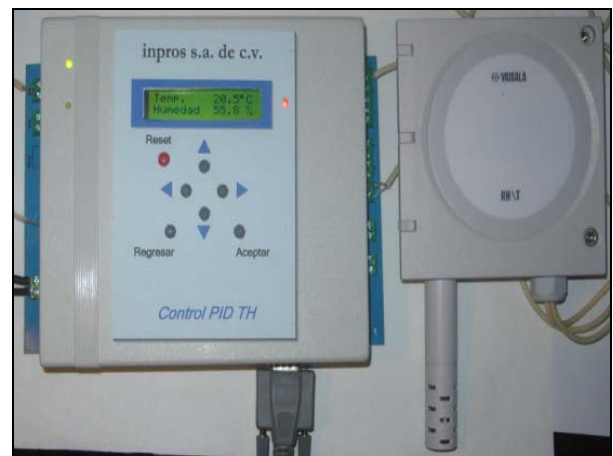
Fig. 16 Controller board and sensor
