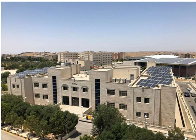
Fig. 4 1MWp TTU PV system for rooftop
