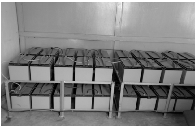
Fig. 4 Battery Bank used for Storage Purpose
