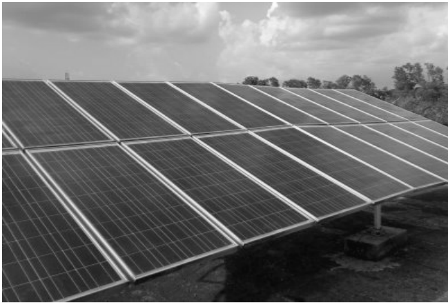
Fig.2 Solar Array of the System under Study
