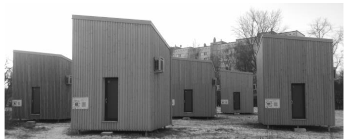
Fig. 1. Experimental test buildings.
