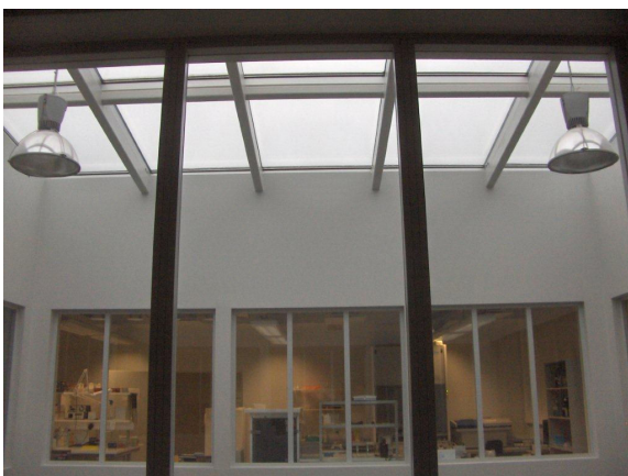
Figure 6. Three-storeyed atrium-type building (C).
