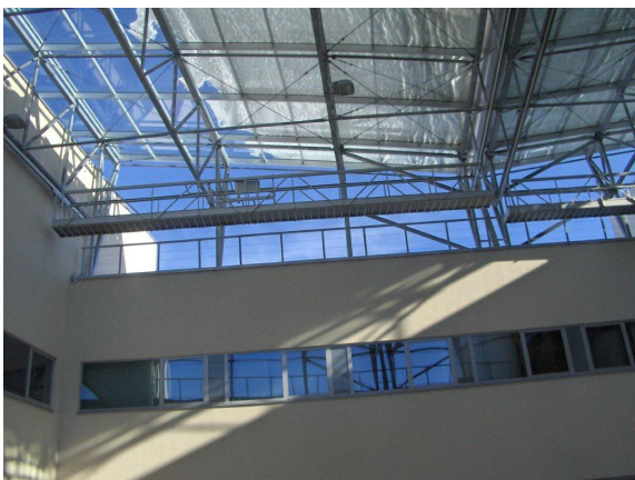
Figure 4. As there is a slot between the roof and walls in the building (B), the snow is falling on the atrium floor in winter.
