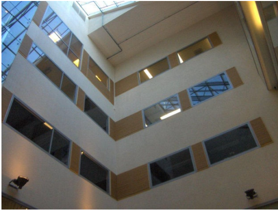
Figure 2. Atrium-type building (A) that is tightly covered with glass roof. Only the workrooms beginning from the 4 th floor are sun-lighted.
