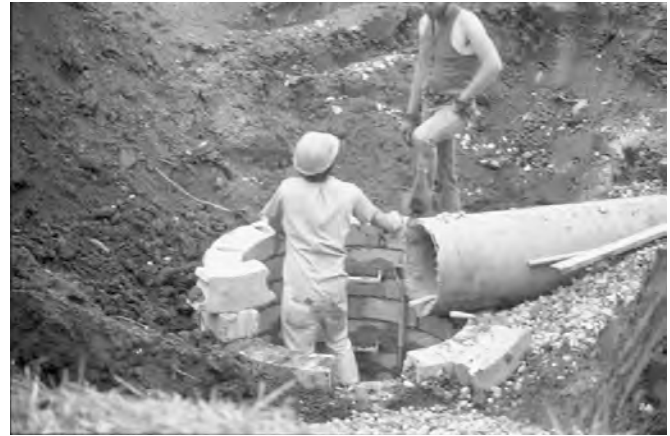
Figure 22. Installation of water conveyance systems (copyright © 1980 Jon Bryan Burley, all rights reserved, used by permission).
