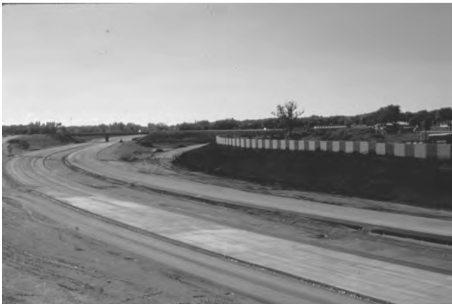
Figure 12. A photograph of the new County Road 18 being built in the early 1980s looking south with Lohman's Amhurst on the right. The organic soils from Auburn were used as fill to create the berm behind the noise wall (copyright © 1980 Jon Bryan Burley, all rights reserved, used by permission)..
