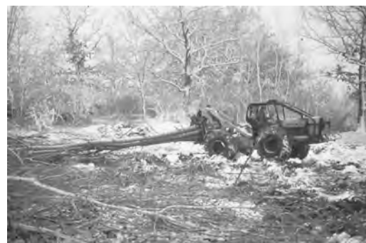
Figure 14. Cut trees were then hauled to a site for chipping. This location in this figure, was the site of one of the detention ponds and had to be excavated early in the process to facilitate site drainage. (copyright © 1979 Jon Bryan Burley, all rights reserved, used by permission).
