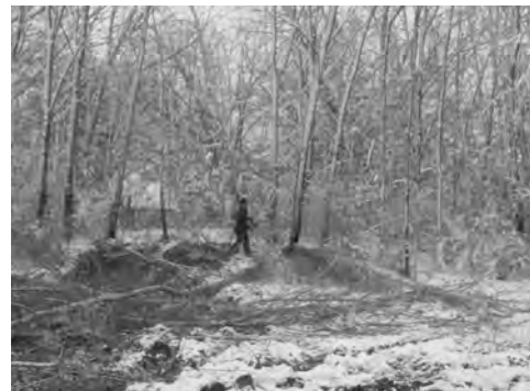
Figure 13. Tree removal at Lohman's Amhurst. Each tree was marked and identified for removal or to remain. Contractors would only cut the trees marked for removal. (copyright © 1979 Jon Bryan Burley, all rights reserved, used by permission).
