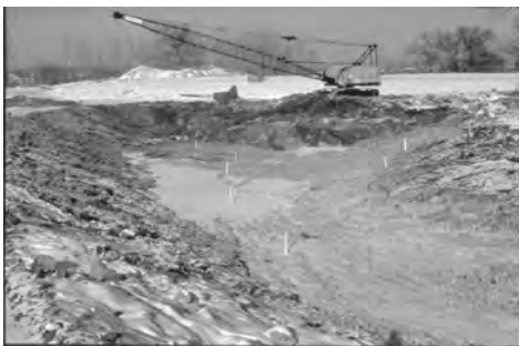
Figure 21. A pond area created to facilitate site drainage. Notice the surveyor's stakes to guide the proper grading elevation of the pond. The pond is made quickly during the non-rainy season and ready to accommodate spring runoff (copyright © 1980 Jon Bryan Burley, all rights reserved, used by permission).
