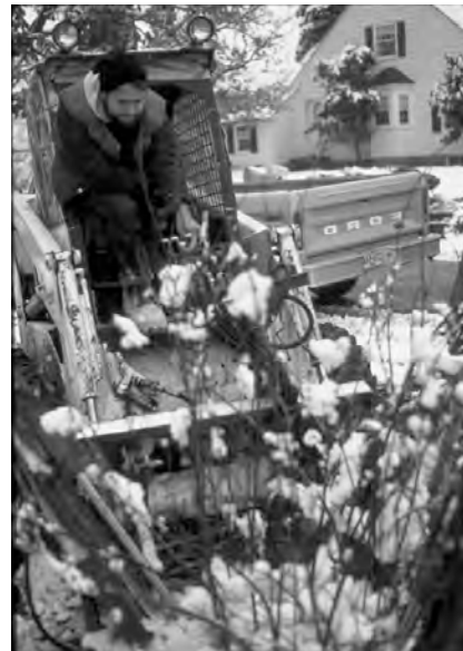
Figure 19. Vegetation from Auburn being installed at Lohman's Amhurst. Single family homes in the background (copyright © 1979 Jon Bryan Burley, all rights reserved, used by permission).
