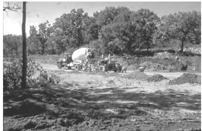
Figure 24. Mid-spring installation of the base gravel course and curbs in preparation for the base asphalt course (copyright © 1980 Jon Bryan Burley, all rights reserved, used by permission).
