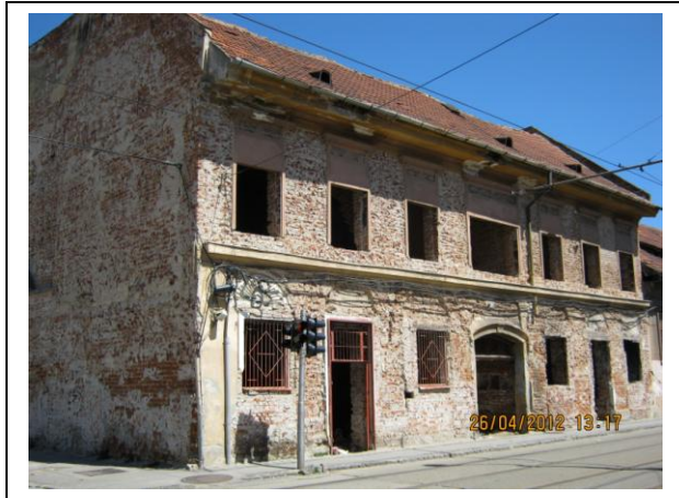
Foto 1 Degradated historical building (Muțulescu 2012)
