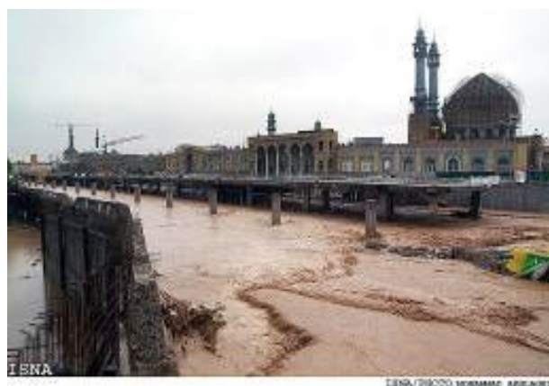
Fig.7a damages in Qom city close to holly place.
