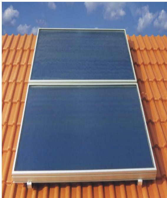
Fig. 2 The solar flat collectors located at roof
