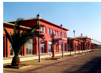
Figure 11 The marina commercial complex – land facilities
