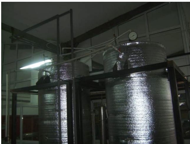
Fig. 3. Front view of the pilot installation [17]
