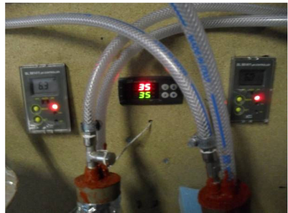
Fig. 9. pH controllers for the small scale installation
