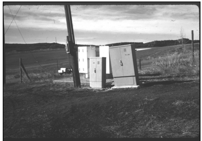
Figure 11. This image of utility pedestals in Colorado was rated by North American respondents as having very poor visual/environmental quality (Copyright 1988 © Jon Bryan Burley, all rights reserved, used by permission).
