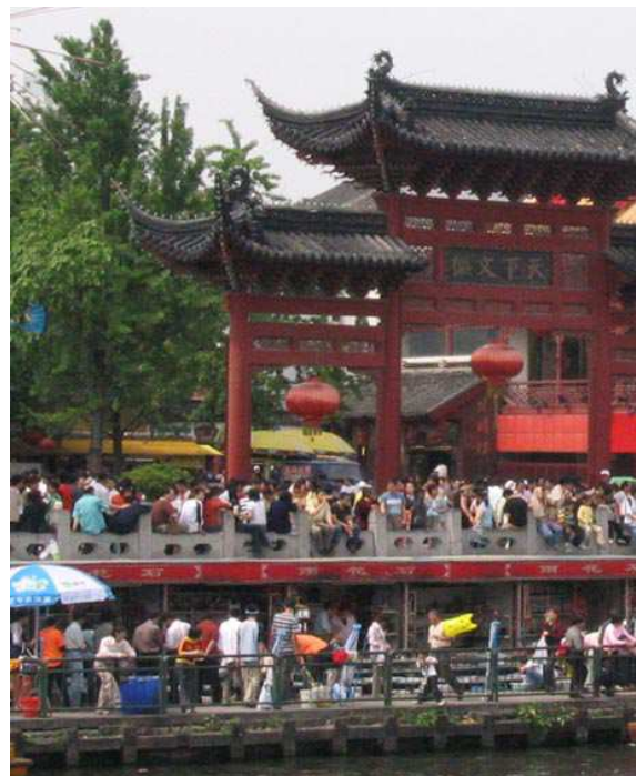
Fig 5 A certain hazard exists to pedestrians when sitting on the handrails. Copyright 2013 JI Jianle, all rights reserved used by permission.
