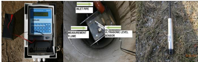
Fig. 5. Measurement devices - Data unit M4016 in shaft A, Measurement flume with ultrasonic level sensor, Pressure sensor LMP307
