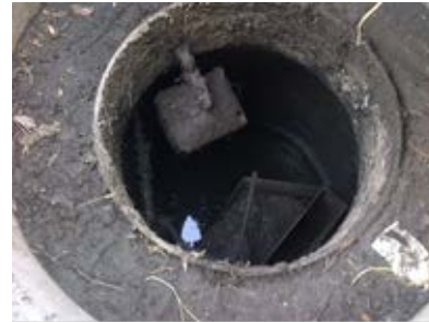
Fig. 18. Flooded filter shaft with measurement devices
