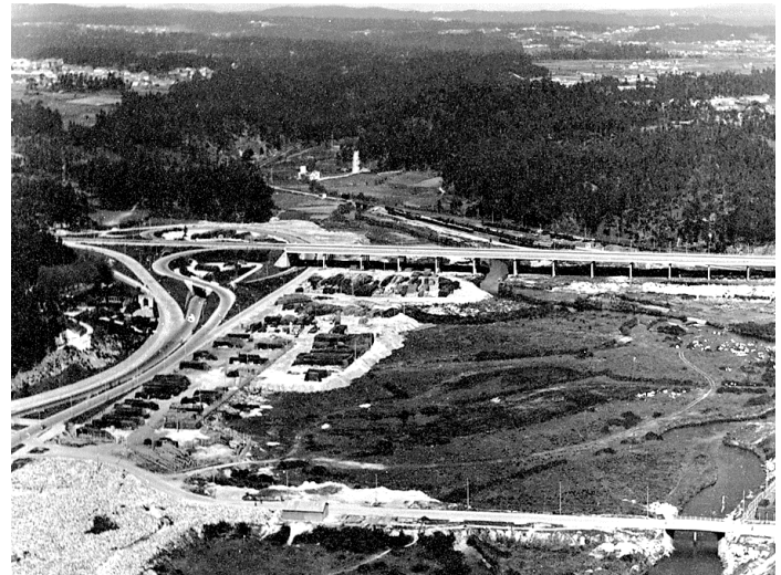
Figure 3. Leixões Harbour. Construction of docks, bridges, buildings and access along 50s, 60s and 70s. Matosinhos (s/d.) Source: APDL
