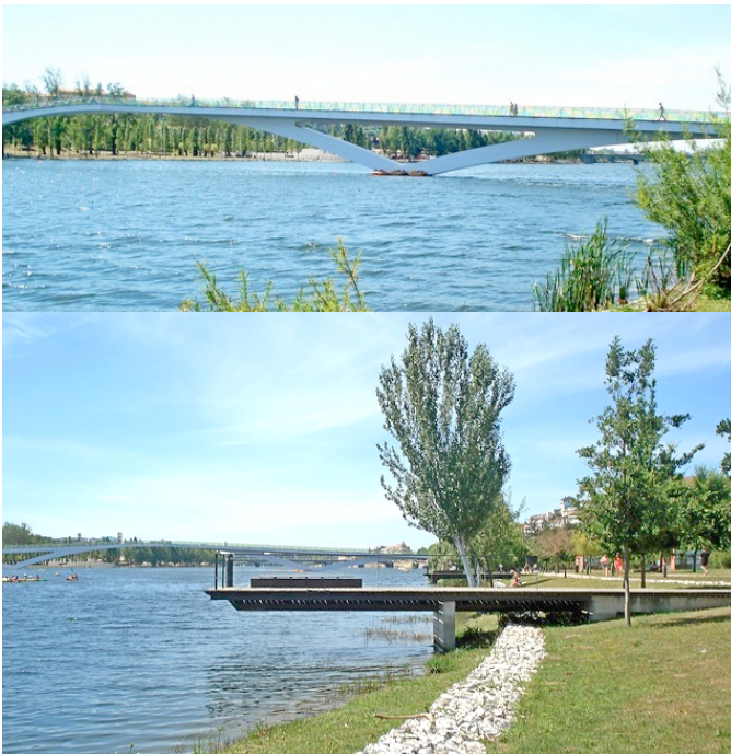
Fig. 7 – “Pedro e Inês” Bridge, zooming out from the right bank margins Image credits: Frederico Meireles Rodrigues 2013.
