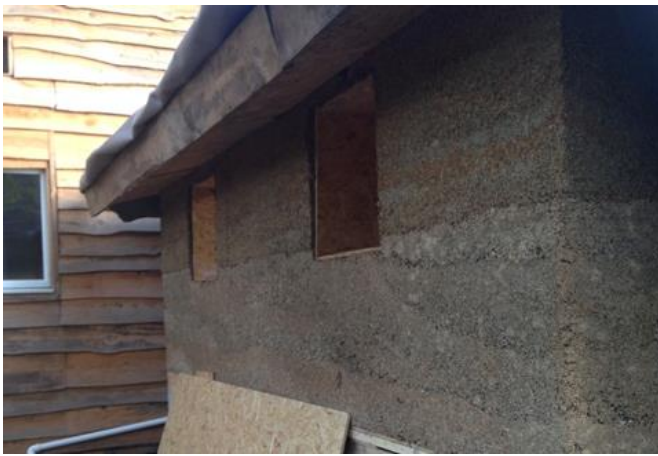
Fig. 11. OSB board struck off at the exterior face of the wall, ready to receive lime rendering
