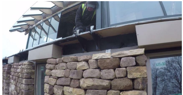
Fig. 3. (a) Site build progress - March 2016
