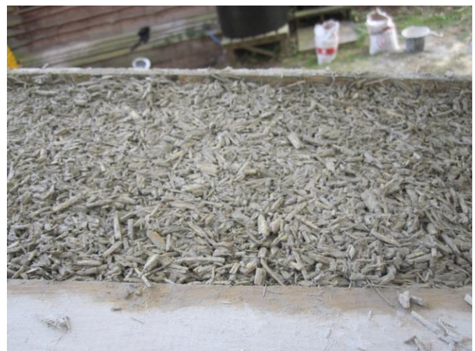
Fig. 10. Hemp wall construction 450mm, with half sycamore half softwood structural timber frame within
