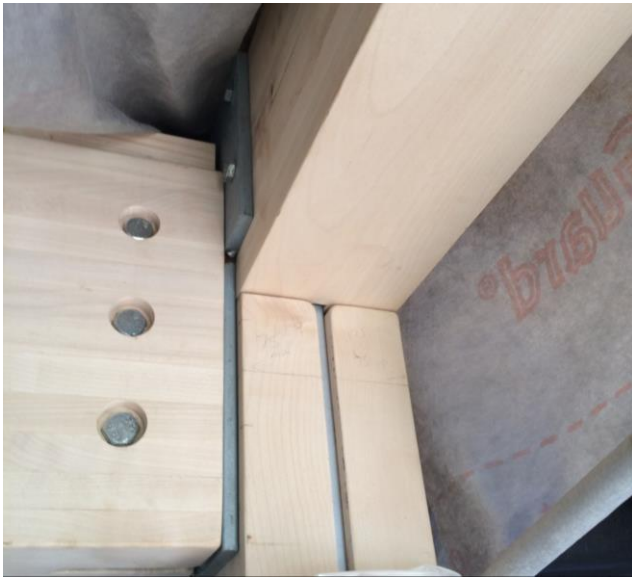
Fig. 17. Fitch Beam – Upper Ground Floor MC =9.5%
