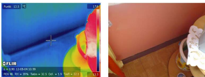
Fig. 7 Thermal bridge formed at the connection of the floor with the external wall exposed thanks to the pressure built up inside the object [10]
