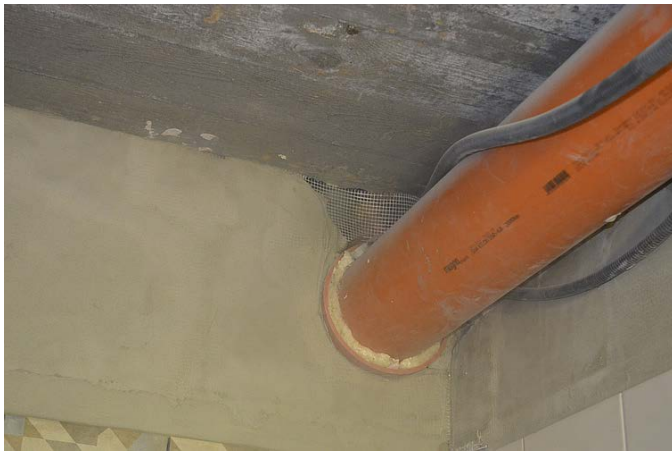
Fig. 11 Leakage caused by improper finishing of the sewage installation cut through the partition [author's own source]
