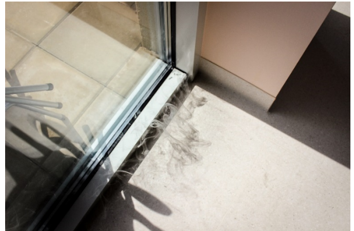
Fig. 13 Sub-pressure conditions, in connection with spot caused smoke on the outside of the building allowed to detect leakages by the observer in the inside. Here: air leakage at the lower edge of the glazed façade
