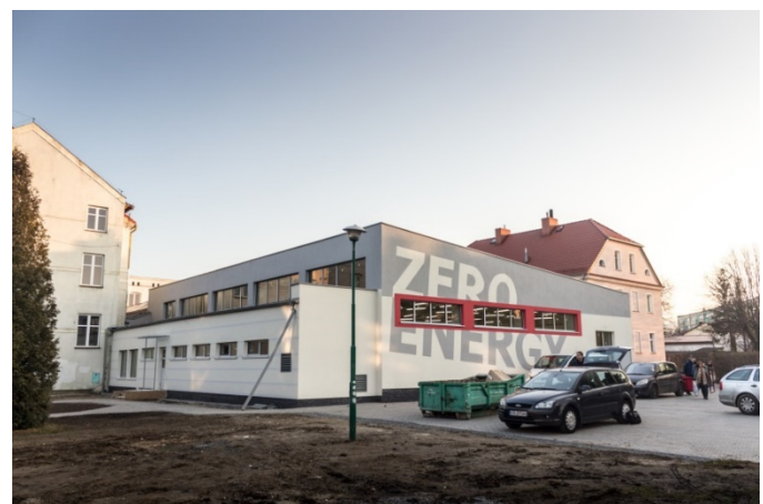
Fig. 16. Low Energy hall in a School Complex of Vocational Education in Bielawa [Source : author's own archive]
