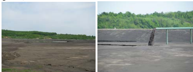
Figure 1. Ceplea Valley ash dump – Branch Electrocentrale Turceni
