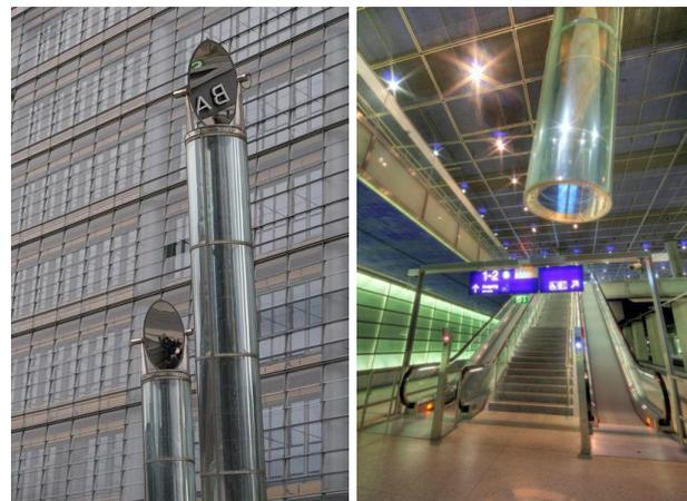
Fig 11. Vertical Light Pipes, Subterranean Train Station
