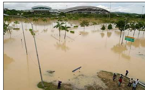
Fig.9. Shah Alam Stadium
