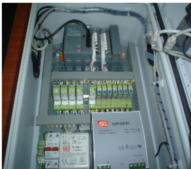
Fig. 9 – Internal view of equipment
