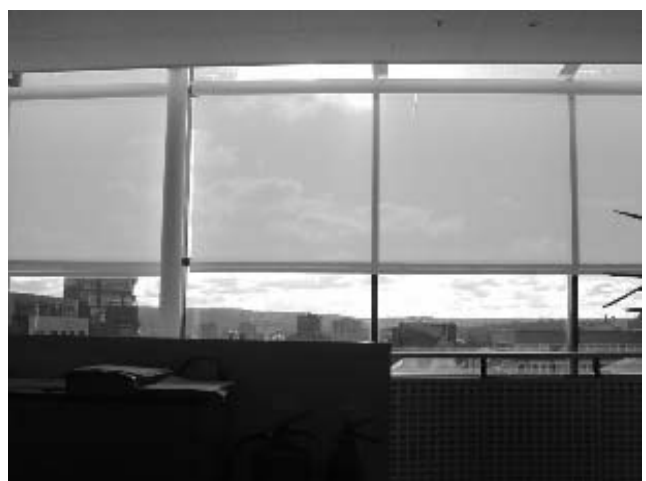
Fig.12 South façade while blinds are 70% closed on a sunny day
