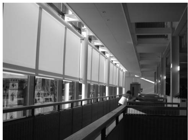
Fig.34 Existing shading of the glazed facade (south orientation) - roller blinds
