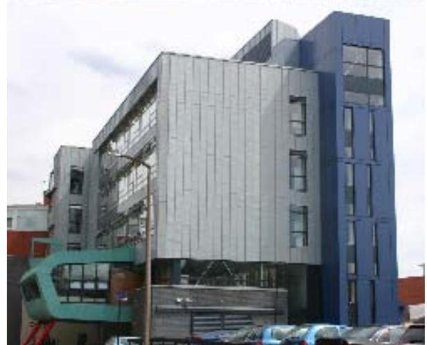
Fig.2 Investigated building ICoSS: south glazed facade with the natural ventilation system (top); northern facade with the main entrance and large windows (bottom)
