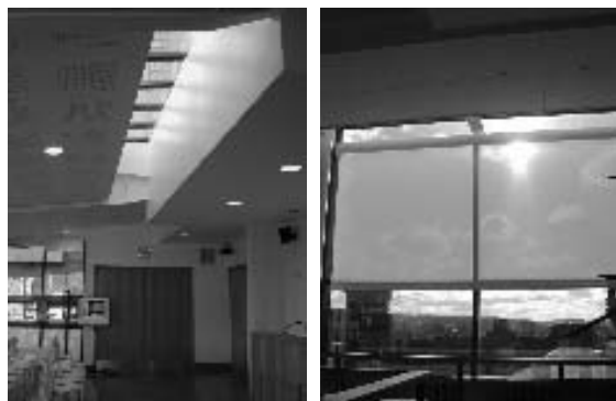
Fig.13 Passive solar design feature (skylight) for maximizing natural daylighting on the north side (left), while preventing sunlight glare effect on the south side (right) during a sunny clear sky conditions
