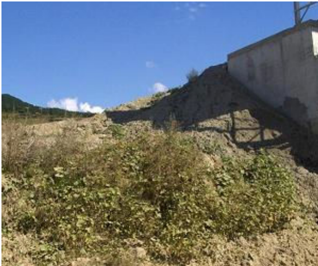
Fig. 3 Deformations, swelling and fractures of the surrounding land filling structure
