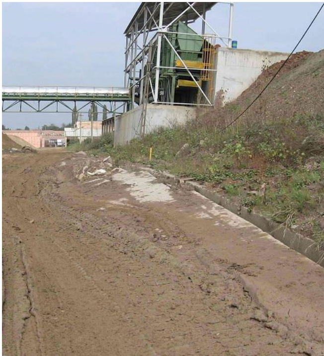
Fig. 15 The access road is deteriorated on a length of about 15 m
