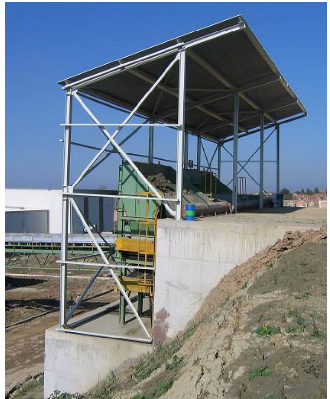
Fig. 10 Side view of the box feeder's structure
