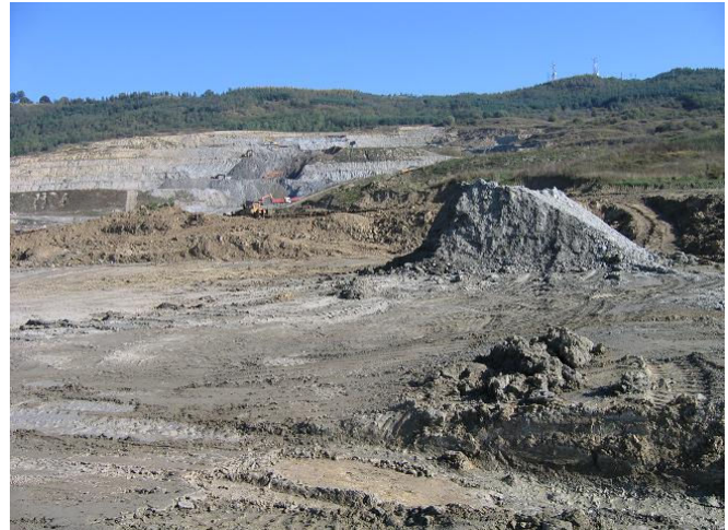
Fig. 16 Amplification of the deformation process due to the possibility of water infiltrations from the proximity slopes
