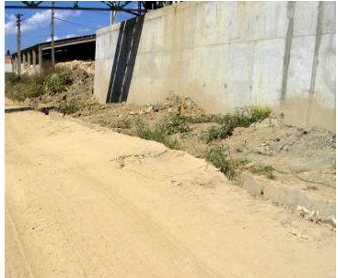
Fig. 4 The soil deformations produced translations and rotations of the structure
