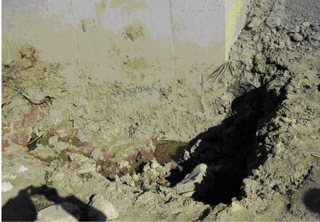
Fig. 8 The survey performed at the foundation of the investigated construction object
