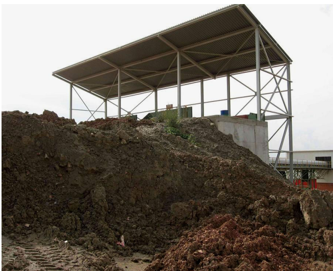
Fig. 9 Construction of the storing platform behind the box feeder
