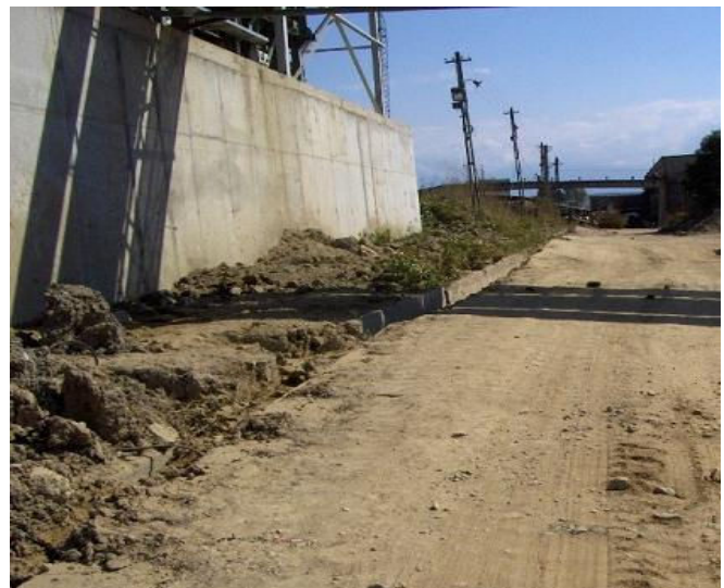
Fig. 5 Soil deformations in front of the structure
