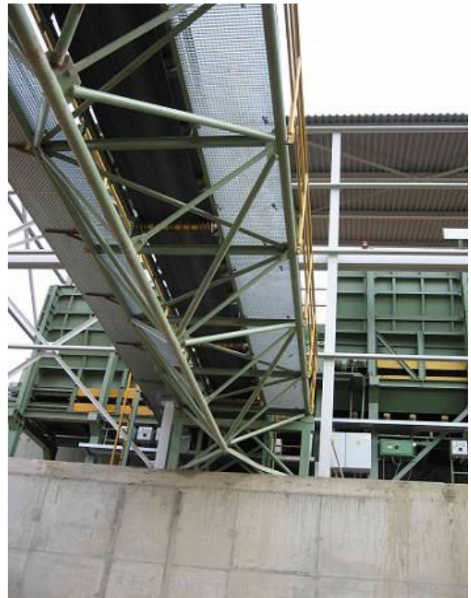
Fig. 7 The box feeder built on reinforced concrete foundation
