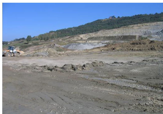
Fig. 2 The storing platform behind the feeder
