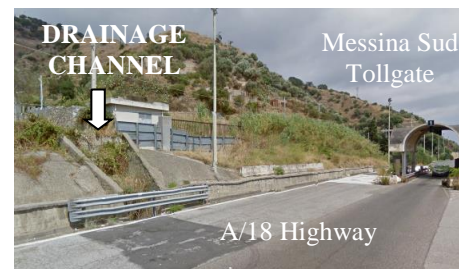
Fig. 5 View of Messina Sud tollgate area of A/18 highway
