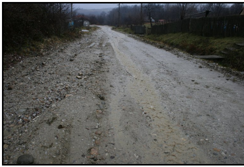
Fig. 12. DJ675C road km 27+000
