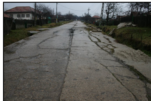
Fig. 11. DJ 675C road km 17+380
