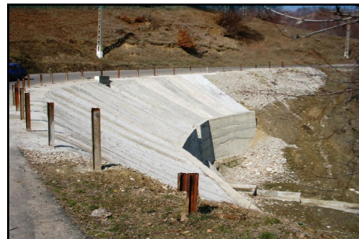
Fig. 19. Consolidation of the road in the degraded area
