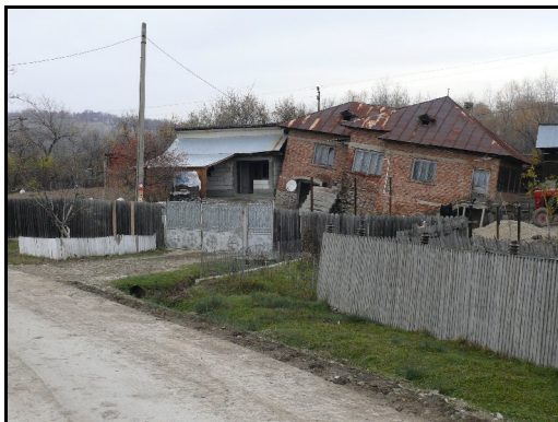
Fig. 15. Aspects of the lignite exploitation impact on buildings in the area
