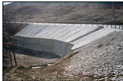
Fig. 18. Retaining wall made of reinforced concrete
