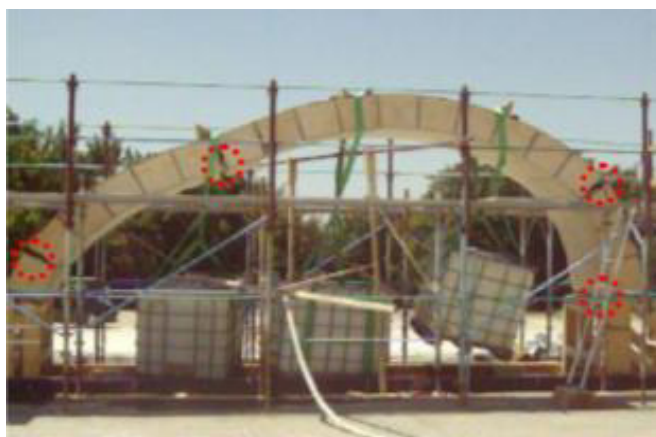
Fig. 4 Collapse mechanism and achievement of the hinges in the arch with an asymmetric load condition.
