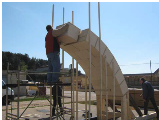
Fig. 2 a) Assembling of the wooden panels to form a closed-form ashlar; b) Assembling of the arch.
