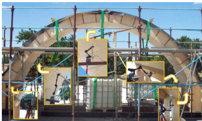
Fig. 3 Tested arch with details of the positioning of the displacement transducers.
