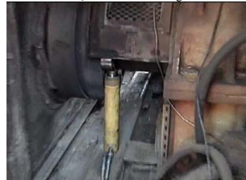
Fig.7) Hydraulic pump for changing rotor position
