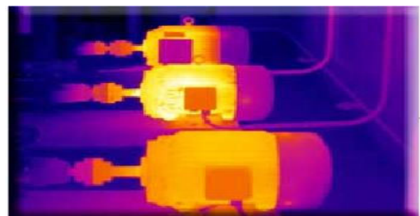
Fig. 10 Overheating at one of the motors at a pump assembly.
