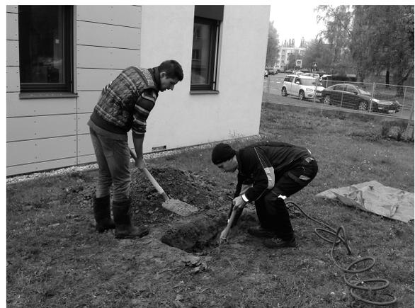
Fig. 3 Installation of ground temperature sensors outside the building
