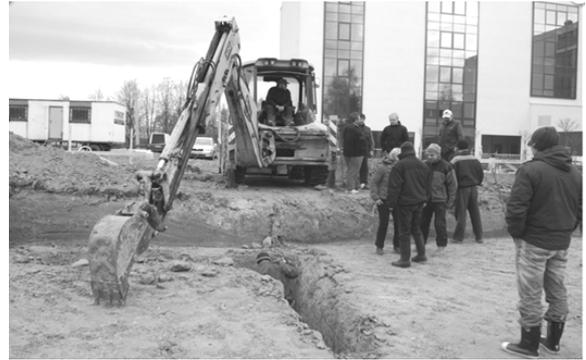
Fig. 2 Installation of ground temperature sensors under the foundation of the building
