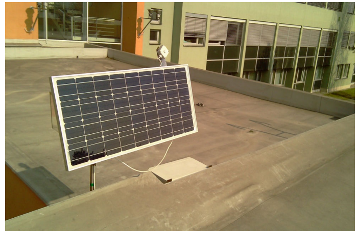
Fig. 2 Photograph of installation of system DE10
