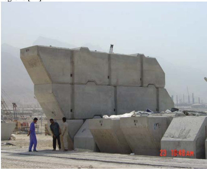
Fig.3 Precast sloping blocks for construction of block work quay wall, Pars Petrochemical Port in Assaluyeh (Iran)
