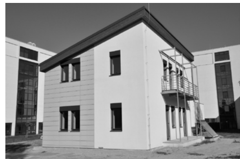
Fig. 1 experimental timber frame passive house (source: RD Rymarov)
