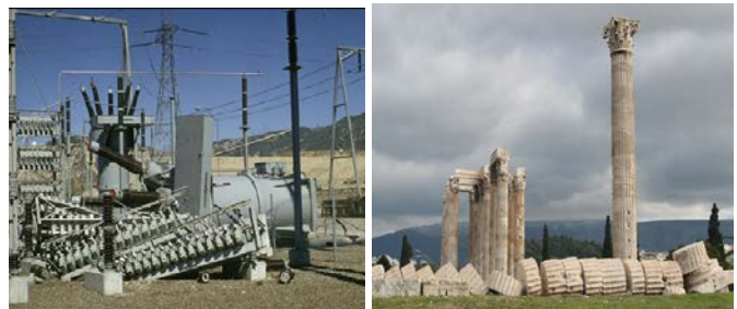
Fig.1: Electrical transformer failure during the 1971 San Fernando earthquake, and remains of the
