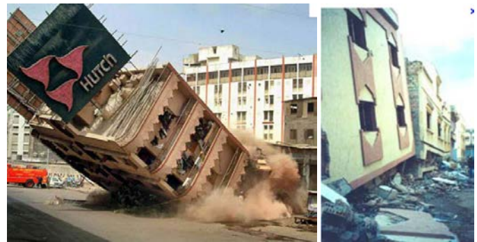
Fig.2: Collapse of soft floors or colonnades.
