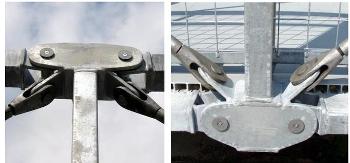
Fig. 4 the pin connections of the upper (left) and lower (right) chords
