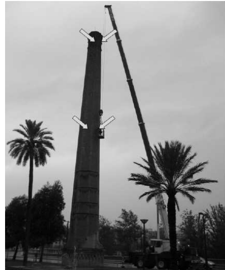
Figure 4: Positions of the accelerometers
