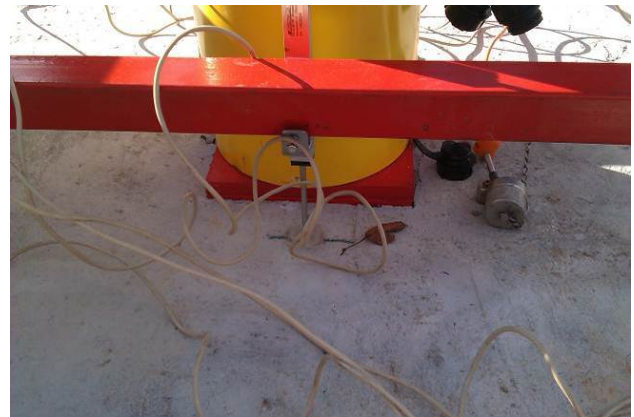
Fig. 13 Punching shear damage under loading area of hydraulic press
