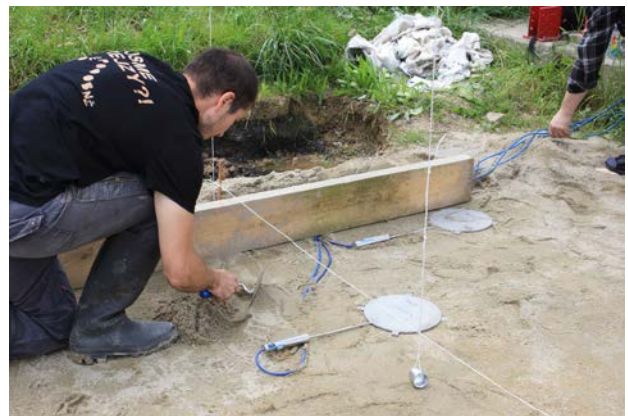
Fig. 5 Installation of geotechnical pressure cells
