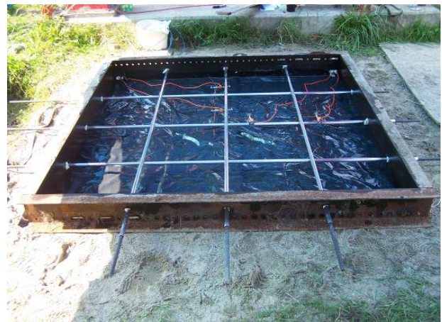
Fig. 1 The steel formwork with ducts for prestressing bars
