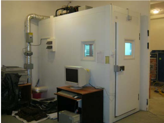
Fig. 6 The air conditioned room
