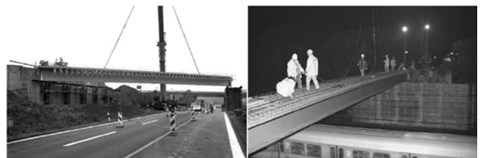
Fig. 5: Bridge using pcb technology crossing existing motorway
