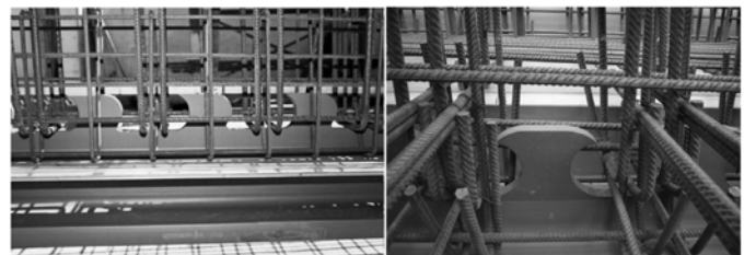
Fig. 14: Examples of reinforcement of composite dowels
