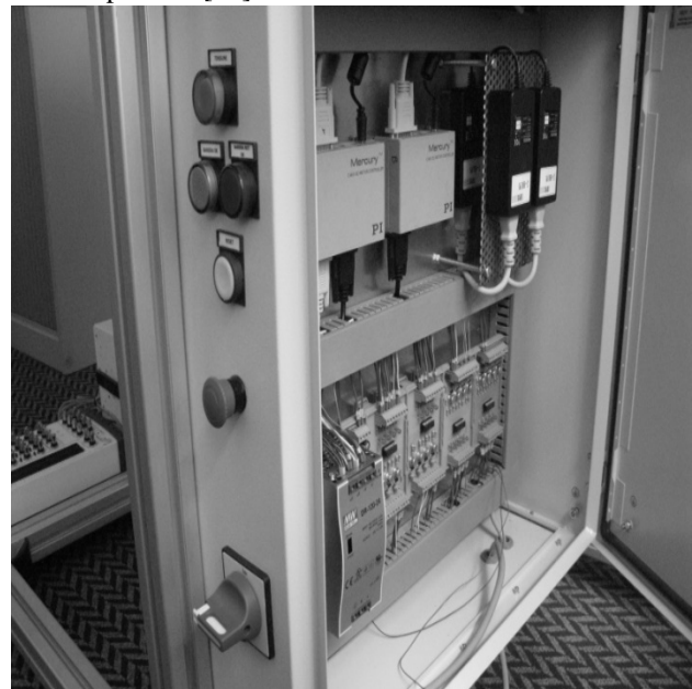
Fig. 1 Electrical control unit
