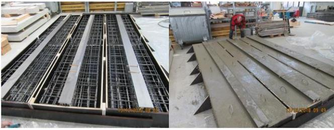
Fig. 9 concreting of the test specimens
