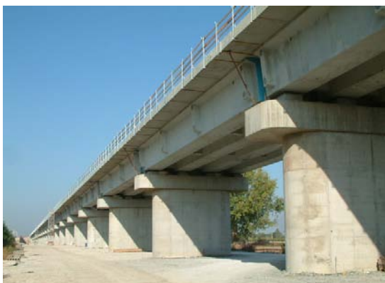
Fig. 2. Lateral view of the sample high-speed railway bridge.
