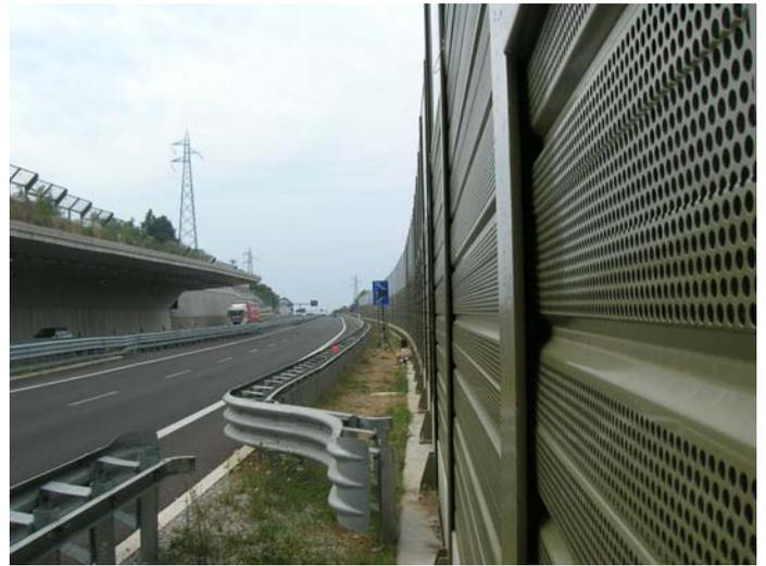
Figure 7 Steel and PMMA barrier
