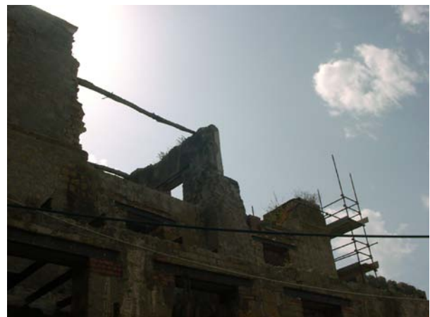
Fig.6 - The exterior of the building embedding the collapsed vaults.
