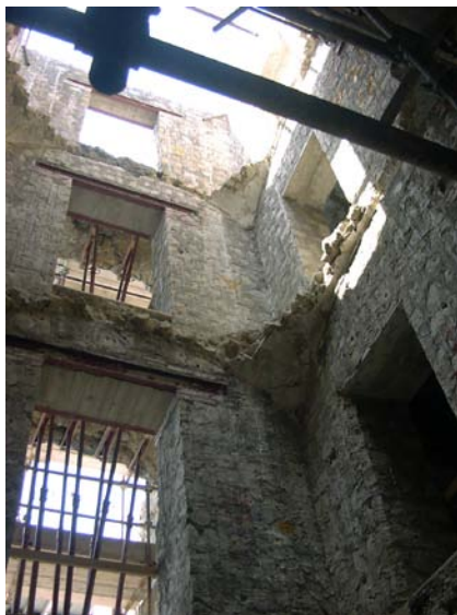
Fig.8 - The standing parts of the building from its interior.
