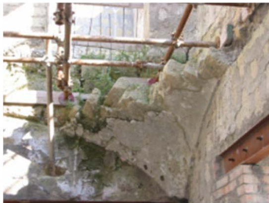
Fig.14 - Detail of the collapsed vault.
