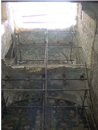
Fig.7 - The standing parts of the building from its interior.
