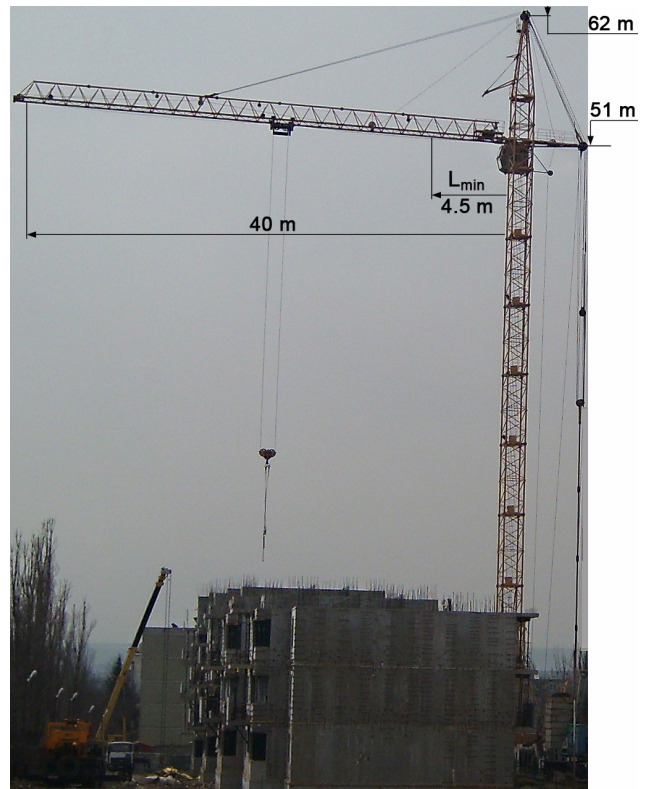
Fig. 3 tower crane KB-408.21 reg.№ 39340 of a loading capacity of 10 t
