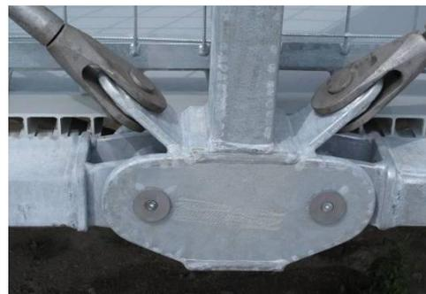
Fig. 6 Structural detailing of assembly joint of truss main girder lower chord of long footbridge
