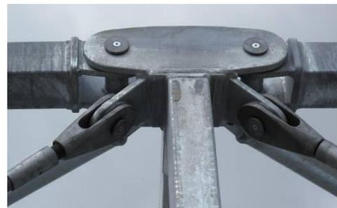
Fig. 5 Structural detailing of assembly joint of truss main girder upper chord of long footbridge
