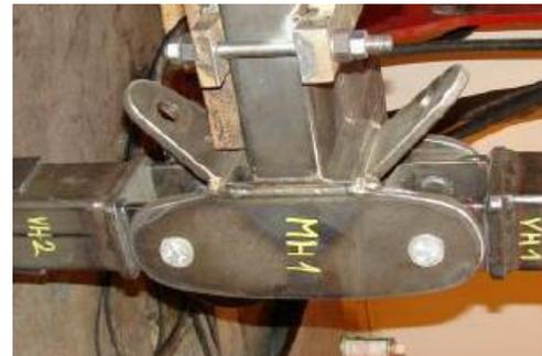
Fig. 11 Illustration of produced assembly joints of long footbridge main girder lower chord
