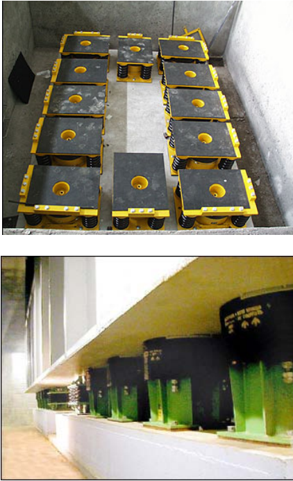
Fig. 3 Mounting viscous-elastic system under technological equipment foundation
