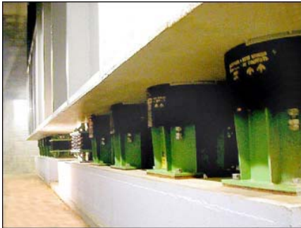
Fig. 3 Mounting viscous-elastic system under technological equipment foundation
