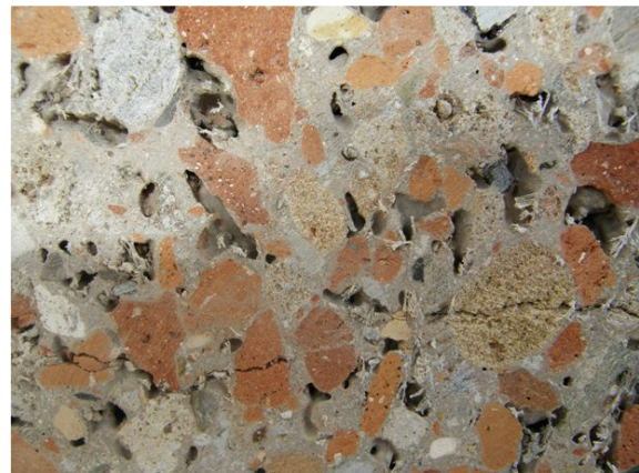
Fig. 9 Grading The porous structure of fibre concrete with masonry rubble
