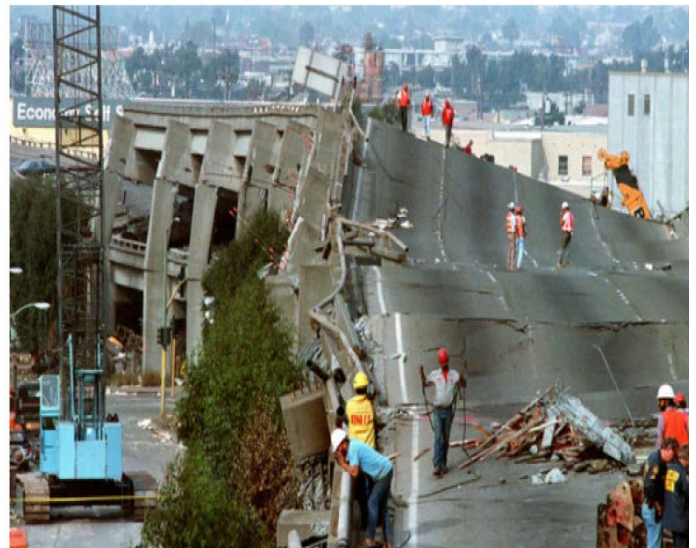
Fig. 3 Failure of Cypress Viaduct Bridge at Loma Prieta earthquake [12]
